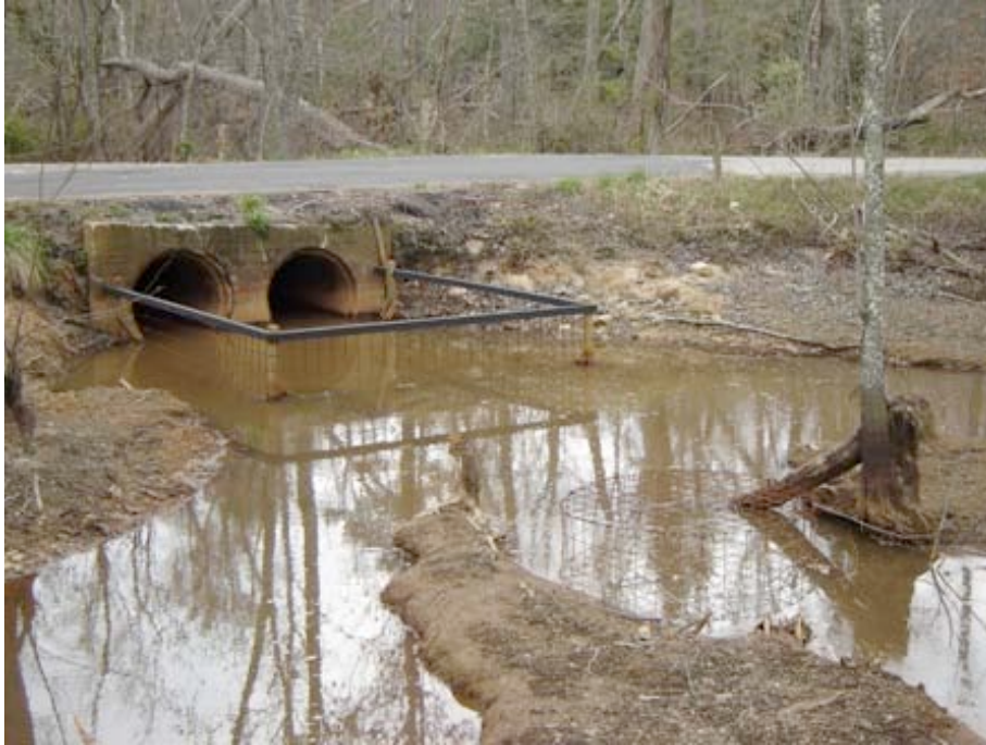
Figure 11. A Beaver Deceiver™ installed in November 2005 to protect two culverts directing water underneath Route 606 on Briary Swamp in Middlesex County, Virginia. A Round Fence™ (bottom center) and a Castor Master™ (beneath the surface of the water between the Round Fence™ and the Beaver Deceiver™) were attached to the upstream end of the Beaver Deceiver™ to augment water flow if beavers attempted to dam the fence.
