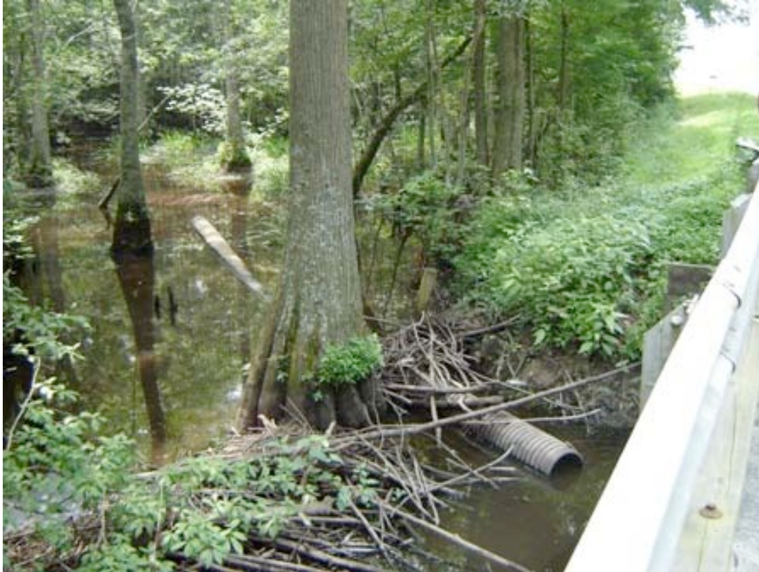
Figure 8. A Round Fence™ (top left) and a Castor Master™ (located beneath the surface of the water between the Round Fence™ and the existing beaver dam) were installed in June 2004 to protect a bridge directing water underneath Route 612 on Corrowaugh Swamp in Isle of Wight County, Virginia.
