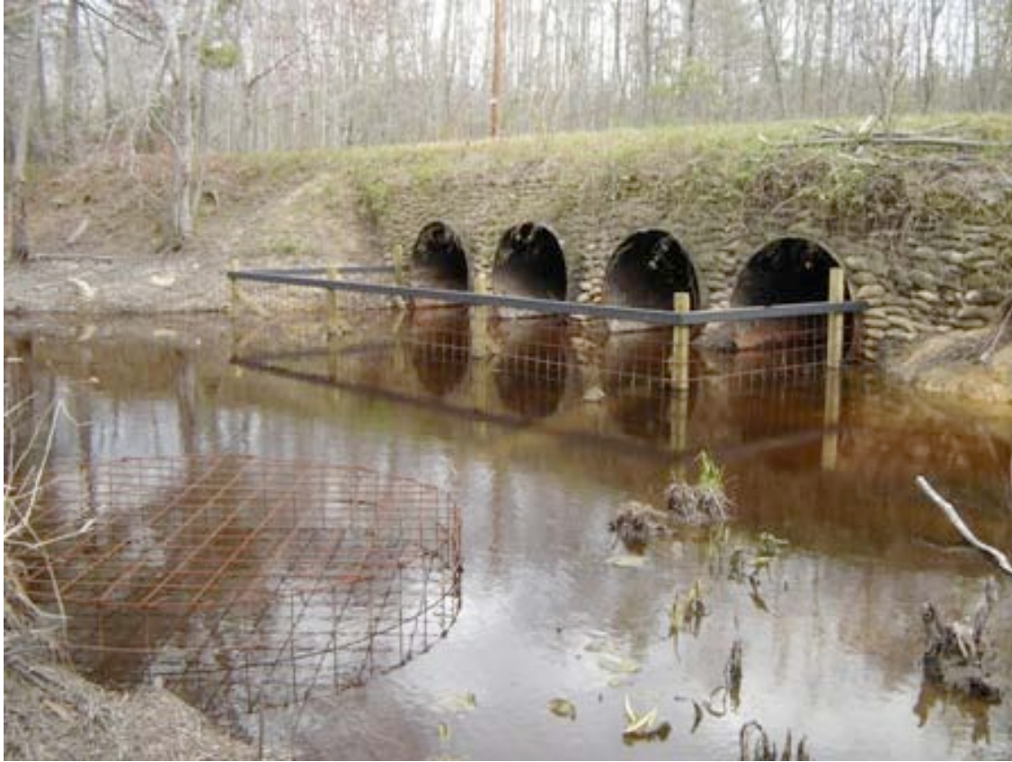
Figure 13. A Beaver Deceiver™ installed in November 2005 to protect four culverts directing water underneath Route 639 on Pope's Creek in Westmoreland County, Virginia. A Round Fence™ (bottom left) and a Castor Master™ (beneath the surface of the water between the Round Fence™ and the Beaver Deceiver™) were attached to the upstream end of the Beaver Deceiver™ to augment water flow if beavers attempted to dam the fence.
