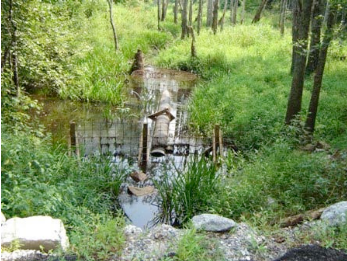
Figure 17. A Round Fence™ (top center) and a Castor Master™ (between the Round Fence™ and the receiver fence) attached to the upstream side of a receiver fence installed in May 2005 to protect a culvert directing water underneath Route 630 on Swift Creek in Chesterfield County, Virginia.
