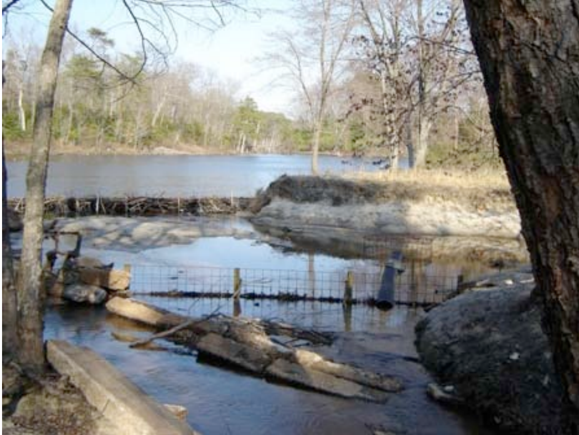
Figure 14. A diversion dam (left center), a Round Fence™ (lower right), a Castor Master™ (lower right) and receiver fence (lower center) installed in November 2005 to protect three culverts directing water underneath Route 616 on Newton's Pond in Westmoreland County, Virginia.
