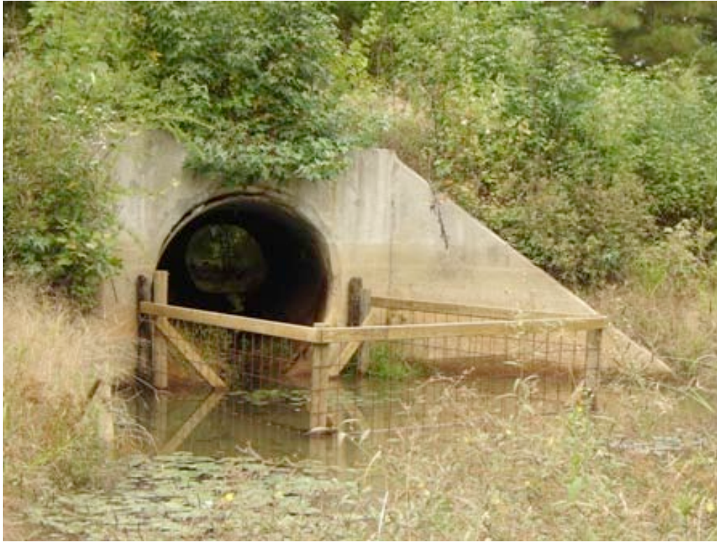
Figure 20. A Beaver Deceiver™ installed in May 2005 to protect culvert directing water underneath Route 1102 on Blackwater Swamp in Prince George County, Virginia.
