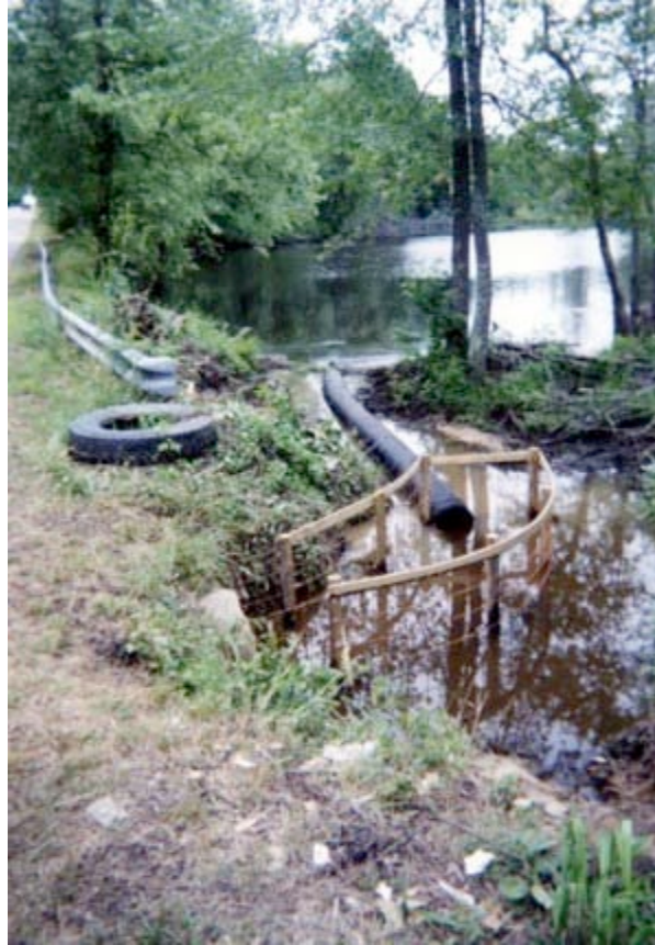
Figure 21. A Beaver Deceiver™ installed in June 2004 to protect a culvert directing water underneath Route 630 on Second Swamp in Prince George County, Virginia. A Castor Master™ (center) and a Round Fence™ (beneath the surface of the water and attached to the upstream end of the Castor Master™) were attached to the upstream end of the Beaver Deceiver™ to augment water flow if beavers attempted to dam the fence.
