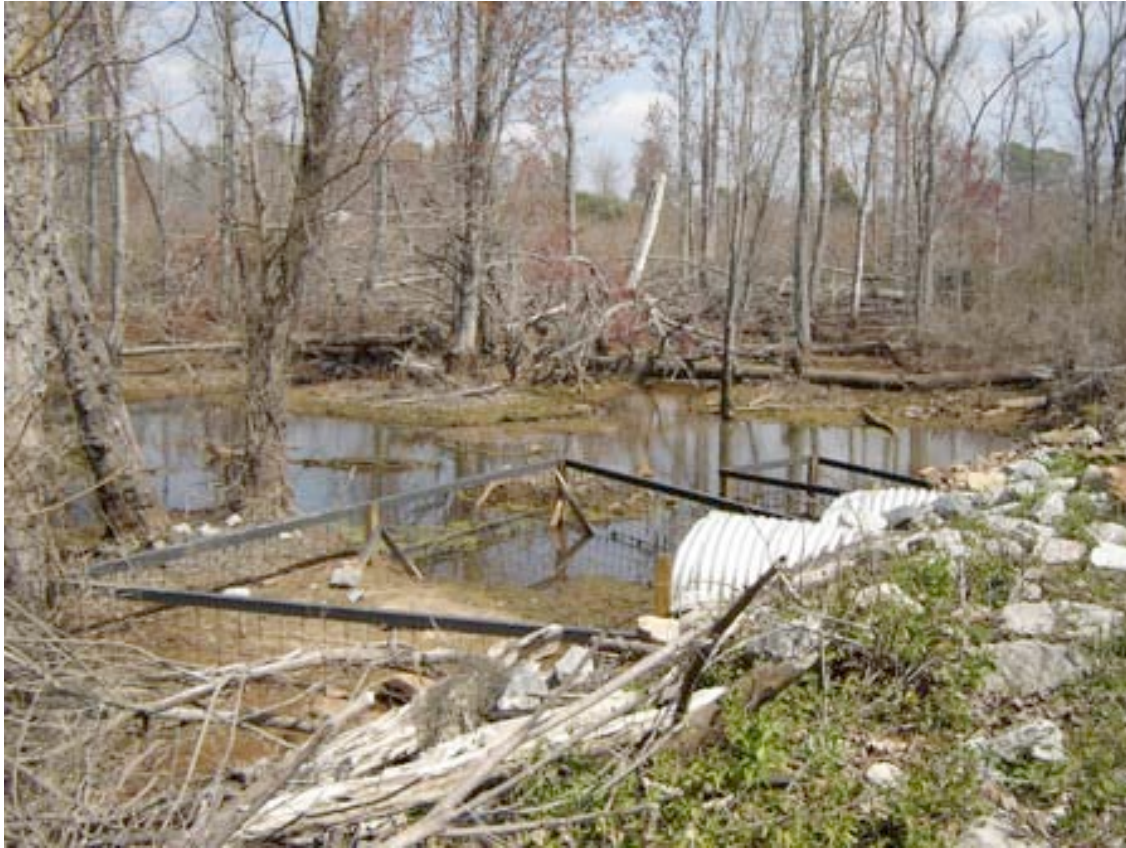
Figure 10. Two Beaver Deceivers™ installed in November 2005 to protect two culverts directing water underneath Route 619 on Craney Creek in Gloucester County, Virginia.
