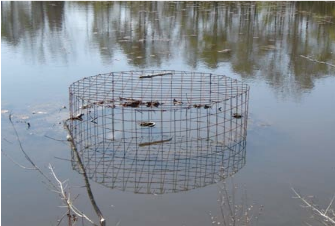
Figure 18. A Round Fence™ (a and b) installed in June 2004 to protect a vertical culvert directing water underneath Route 1102 on Blackwater Swamp in Prince George County, Virginia.
