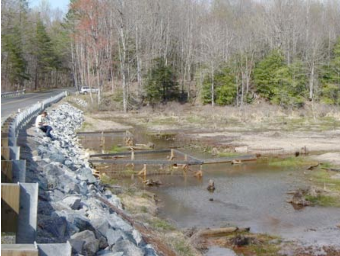
Figure 12. Two Beaver Deceivers™ installed in January 2005 to protect two culverts directing water underneath Route 624 on Pope's Creek in Westmoreland County, Virginia. A Round Fence™ (right center) and a Castor Master™ (between the Round Fence™ and the large Beaver Deceiver™) were attached to the upstream end of one Beaver Deceiver™ to augment water flow if beavers attempted to dam the fences.
