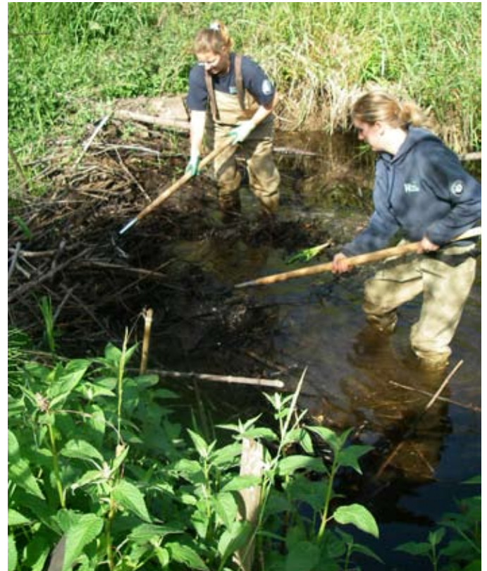
Two interns make a notch in a dam for a flex pipe.
